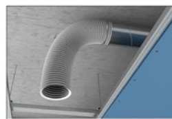
3. Connection to flexible duct pipe
